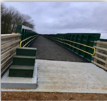
Pic 1 showing ramp +mounting steps
